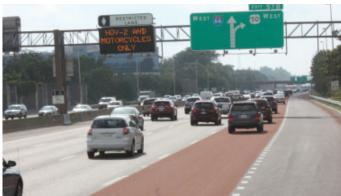
The Virginia Department of Transportation's prime contractor selected DBi Services to install a red colorized high friction surfacing treatment on Interstate 66, west of the Interstate 495 Beltway near Washington DC. This was the first large-scale colorized demarcation pavement project completed in the US for a highway agency.
